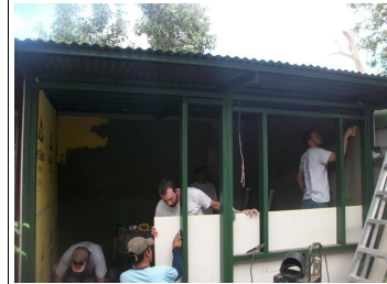
Building the new clinic in Managua
